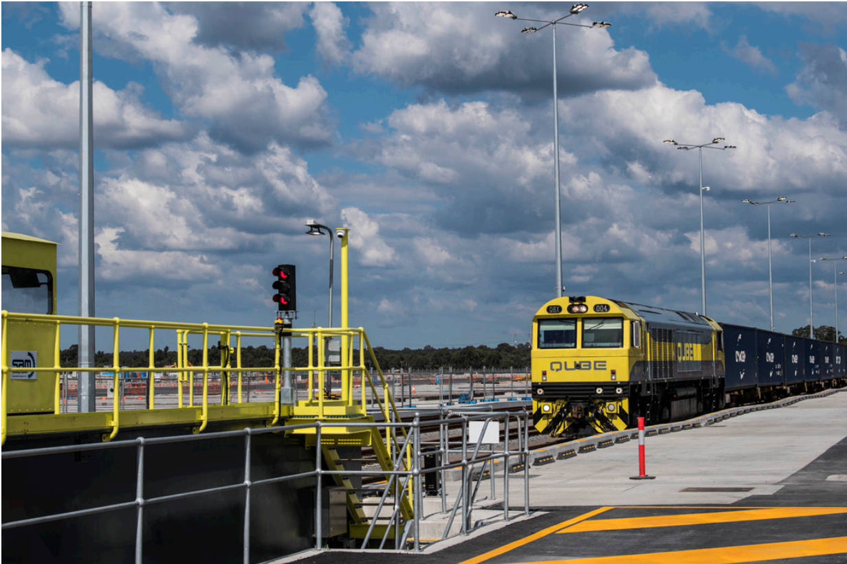
Figure 5: A rail shuttle carrying containers arriving at Moorebank from Port Botany
