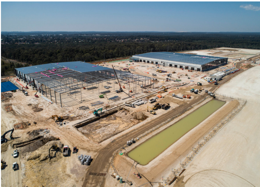
Figure 4: Progress on the construction of warehousing on MPE
