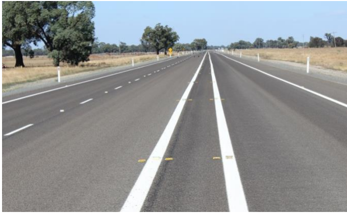
Wide centre line and shoulders on the Newell Highway in southern NSW
