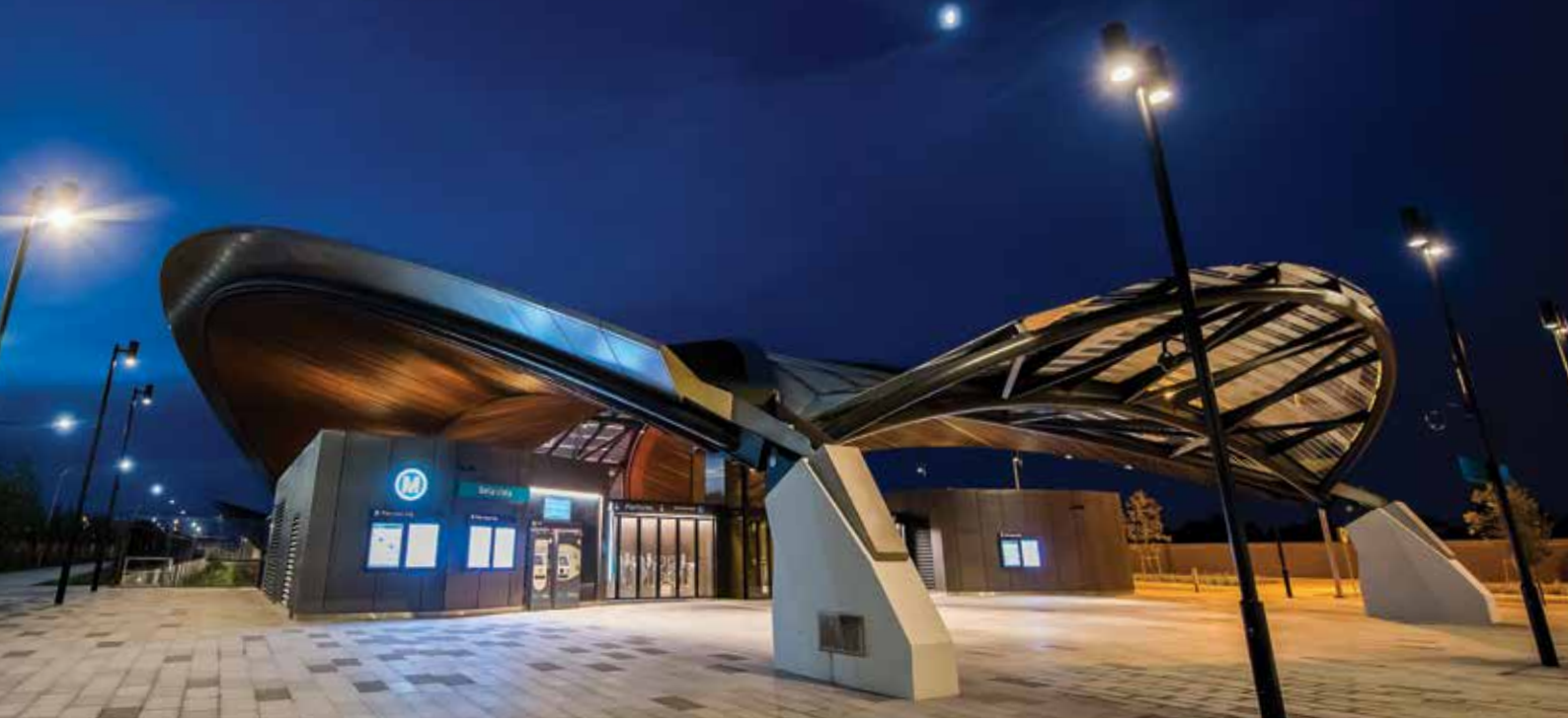
Bella Vista Station, photograph courtesy of Sydney Metro.
