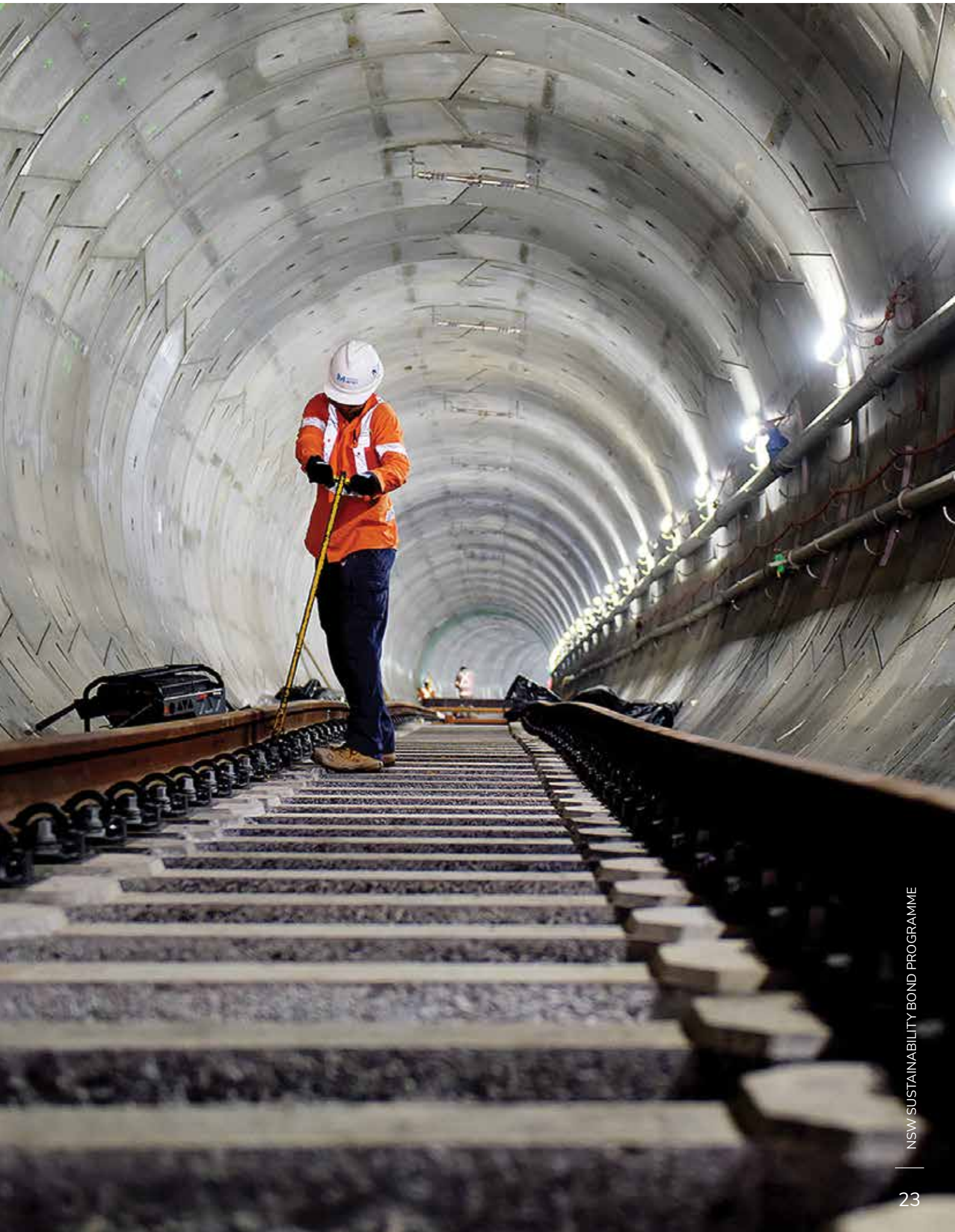
Underground track laying on Sydney's new Metro North West Line, photograph courtesy of Sydney Metro.
