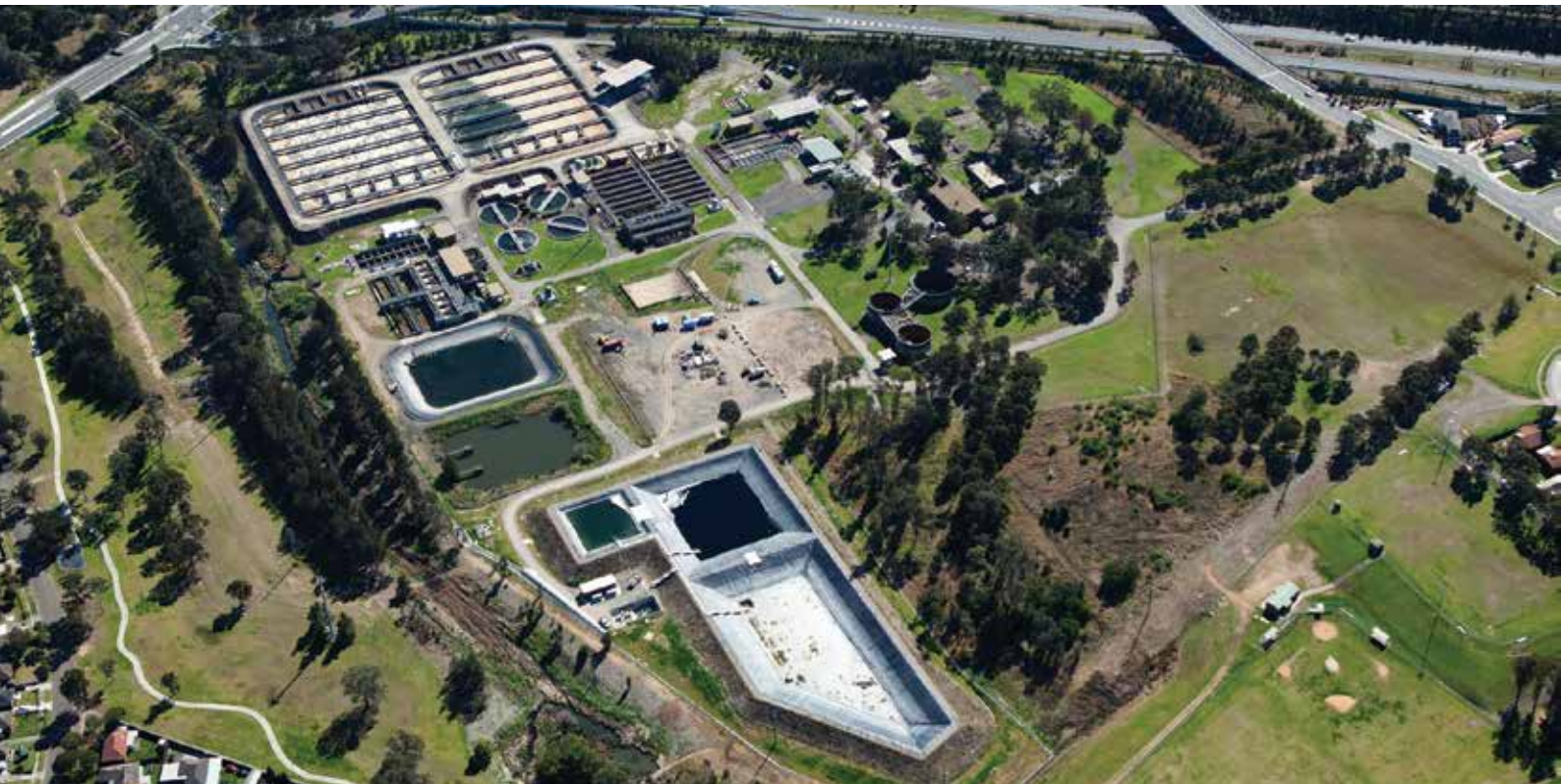
Lower South Creek Treatment Program, photograph courtesy of Sydney Water.
